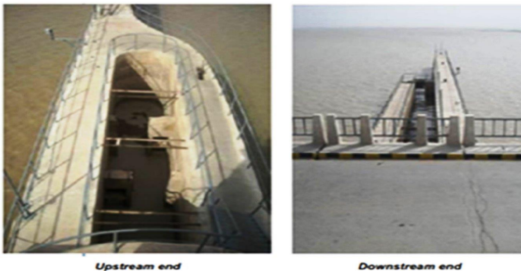
Figure 3 Right side fish ladder at Guddu Barrage (Gate 7)
